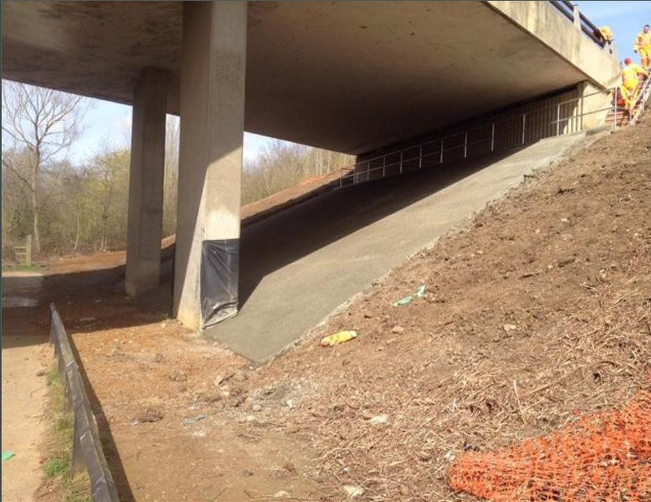
After a number of failures of the slope underneath a road bridge, a contract was let to F J Morris by Milton Keynes Council to repair the revetment.
